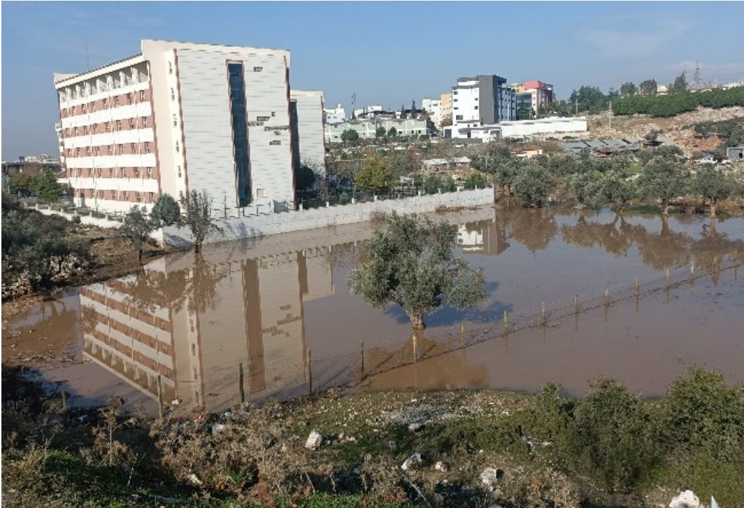
Photo 3. View of the dormitory building built in the Armutlu stream and the accumulated water.
