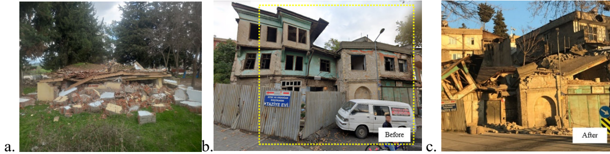
Figure 3. a. Extensive collapse of brick masonry school in Gaziantep b. Historical residential building in Kahramanmaraş before the earthquake sequence and c. After the earthquake sequence.
